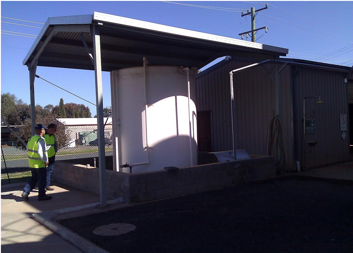
Figure 4.2 - Photo ACH Tank and Bund
