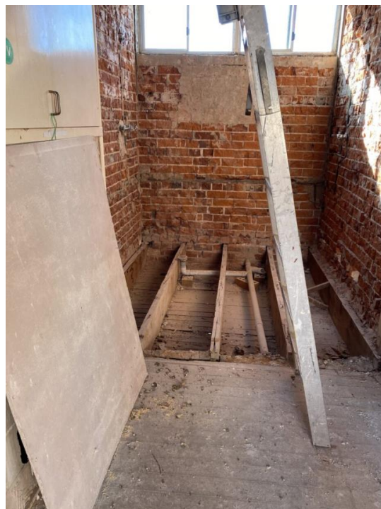
Figure 6.2.4 Timber floor separating storey's when viewed from the first floor.
