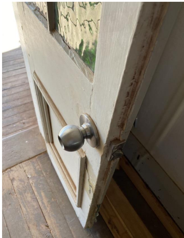
Figure 6.3.3 Example of cylindrical door hardware to be replaced.
