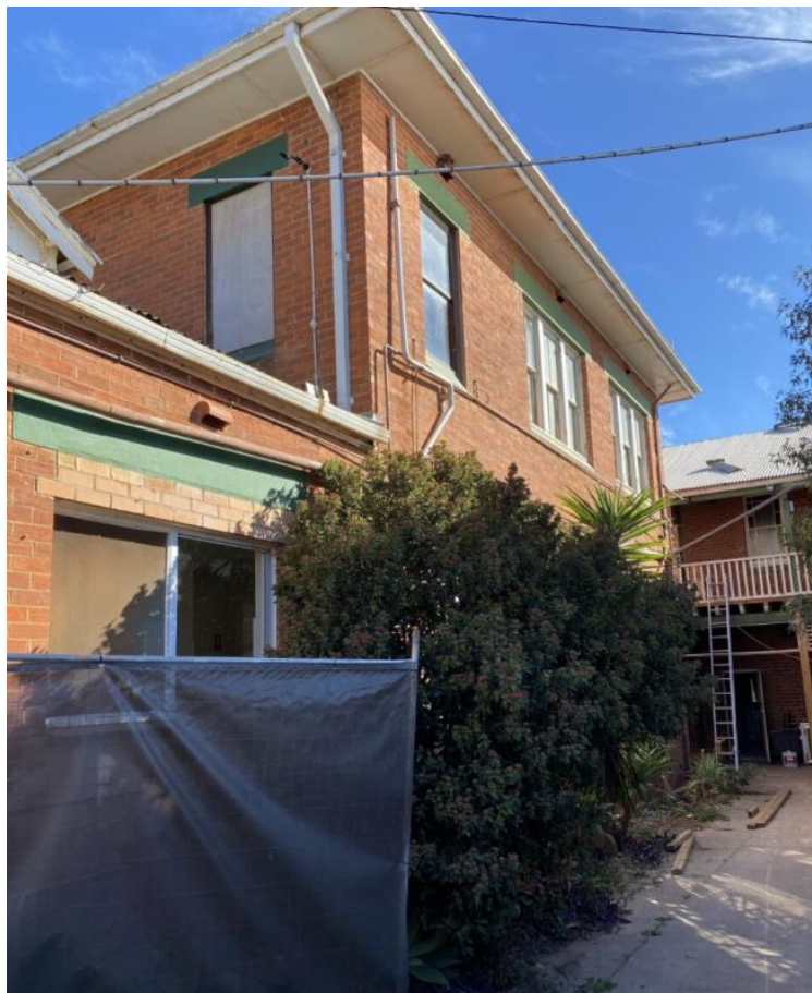
Figure 6.2.1(a) External masonry walls to rear kitchen and managers quarters.
