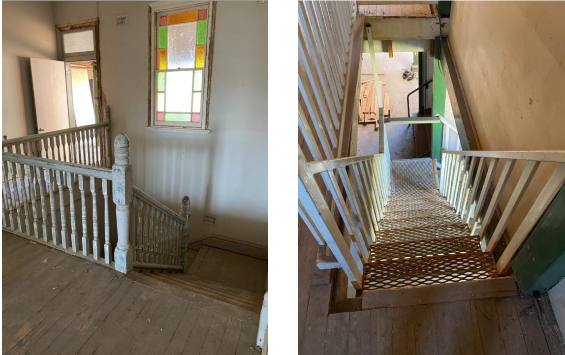
Figure 6.3.2 Existing internal stairway and one of the external stairs.
