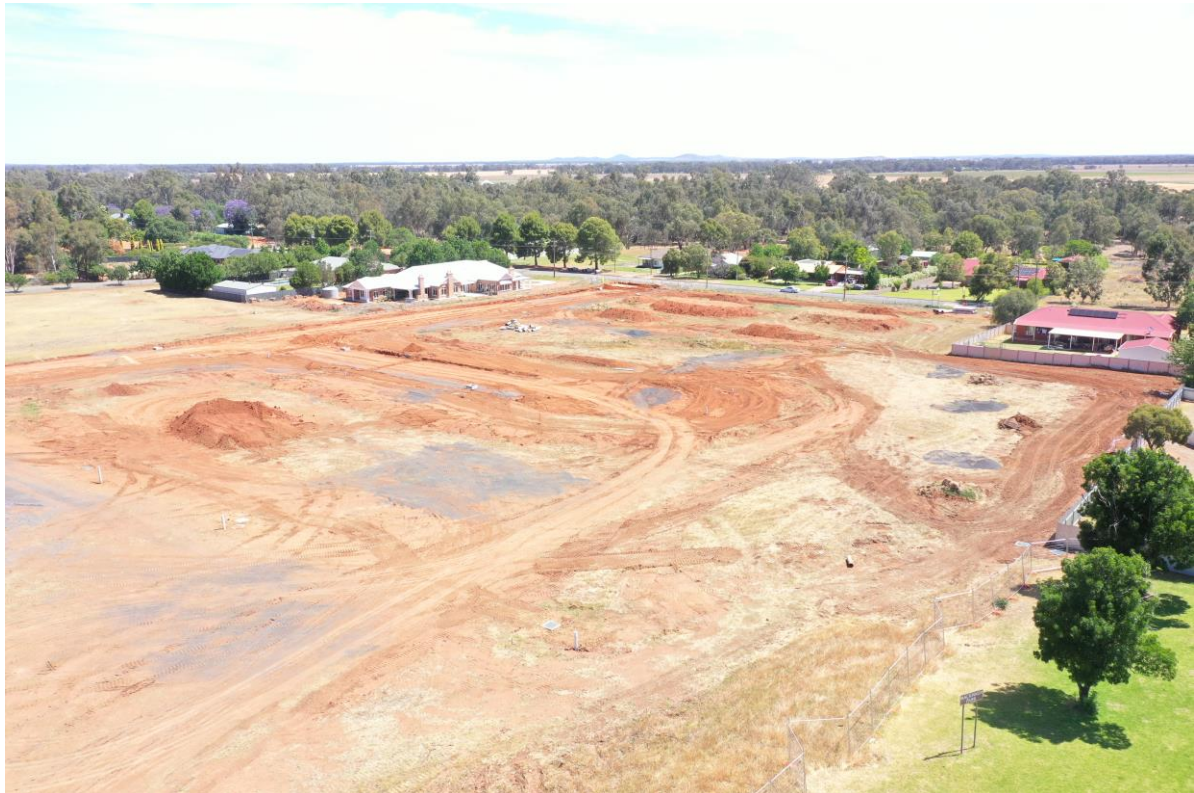
Figure 6 Subdivision Work, Scott Street Condobolin
