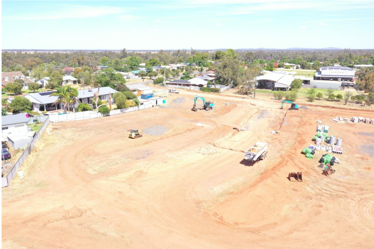
Figure 5 Subdivision Work, Scott Street Condobolin
