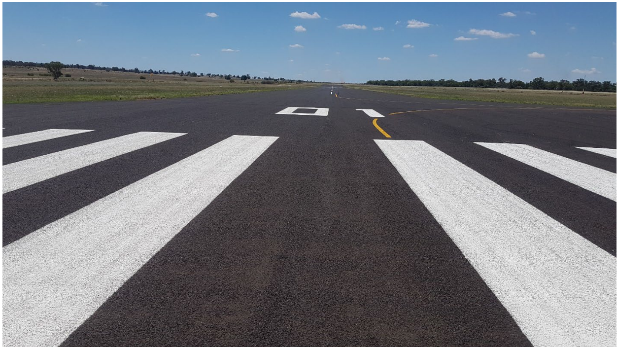
Figure 1 View of Condobolin Airport Runway 01
