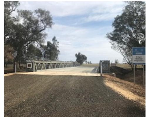
It is a 35m long modular bridge with prefabricated steel truss structure and reinforced concrete abutments.
